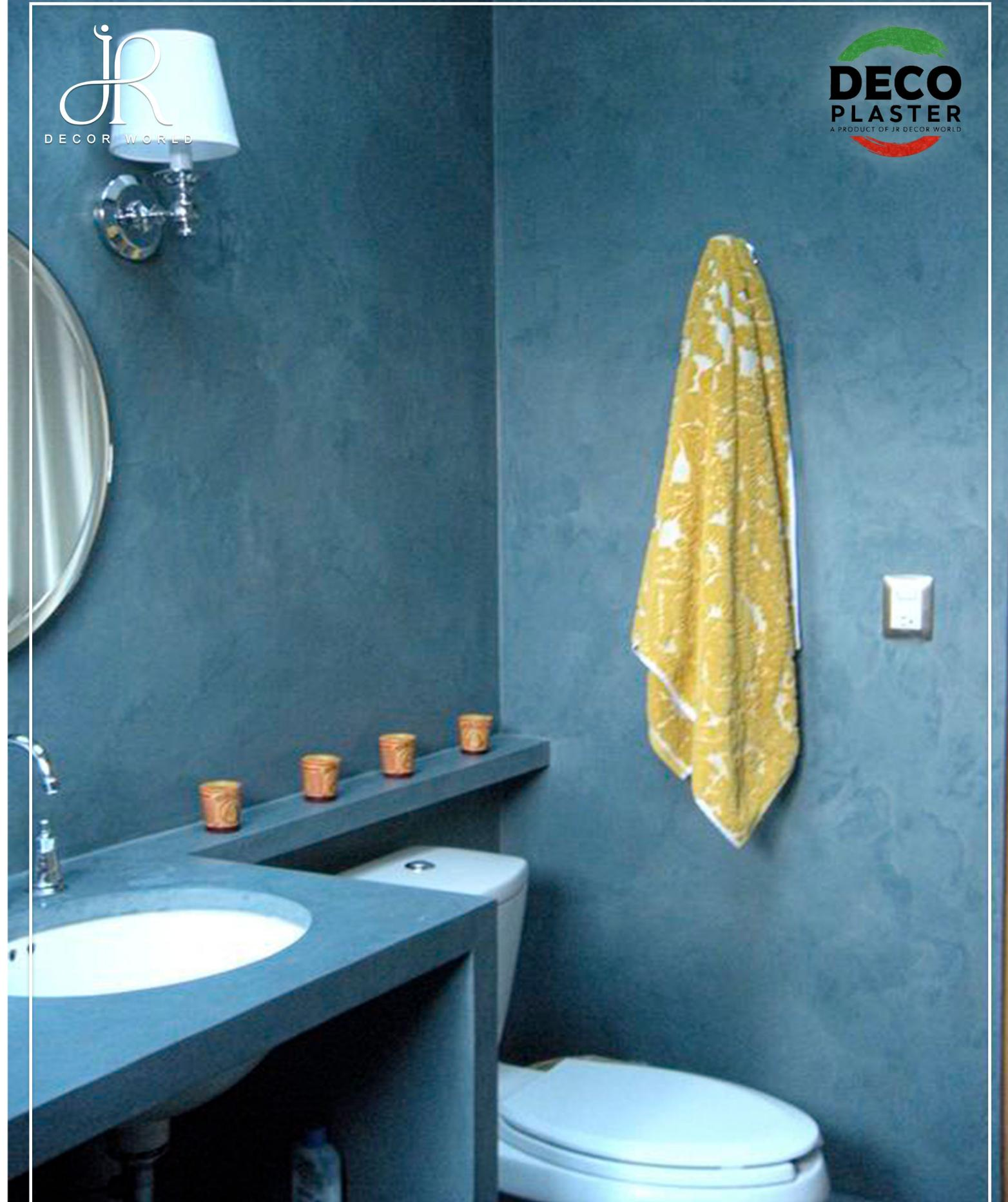
Microcement is a decorative coating composed of cement, water-base resins, additives and mineral pigments that can be applied on a multitude of vertical and horizontal surfaces thanks to its great adhererence.
